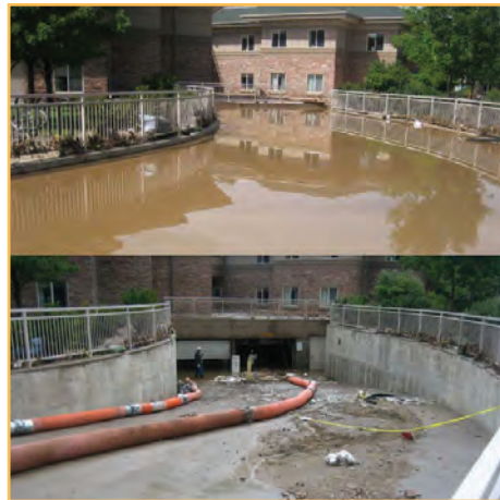
Frasier Meadows garage entrance flooded and during cleanup
